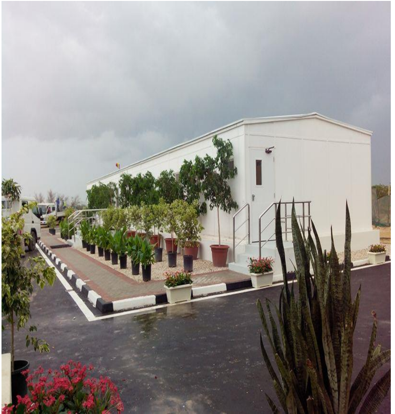
ENGINEERING, PROCUREMENT, INSTALLATION AND COMMISSIONING (EPIC) FOR PORT-A-CABIN AT CONSERVATION AREA IN RAS LAFFAN INDUSTRIAL CITY FOR QATAR PETROLEUM.
