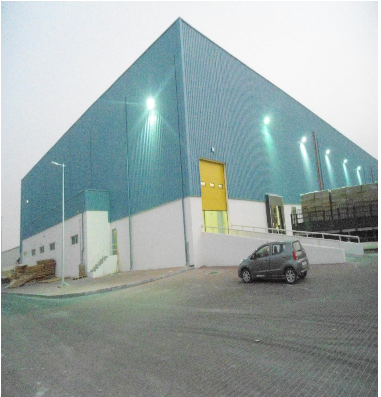
SUPPLY, FABRICATION AND ERECTION OF MEZZANINE FLOOR AT LVQ FOR GULF WAREHOUSING COMPANY
