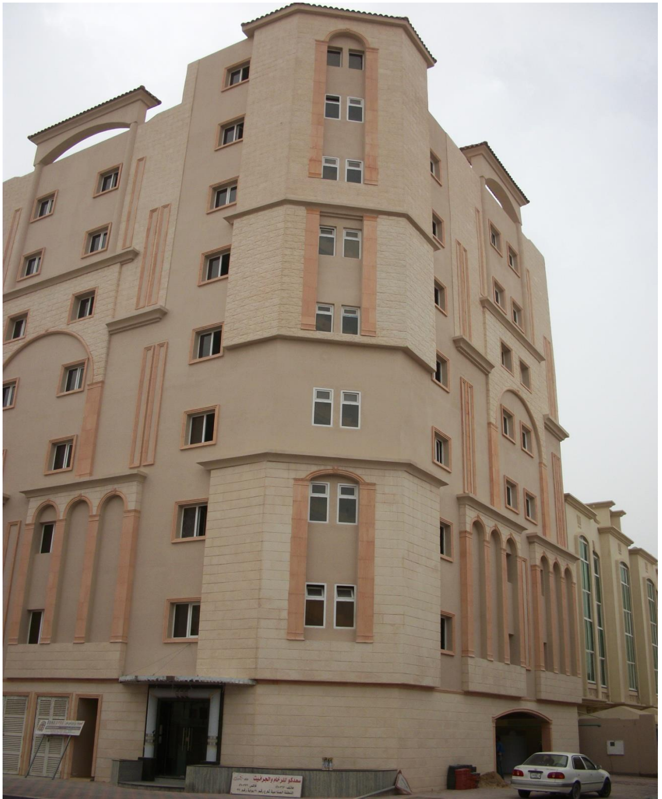
Construction of G+M +6 at Muntazah for Ezaj Management
